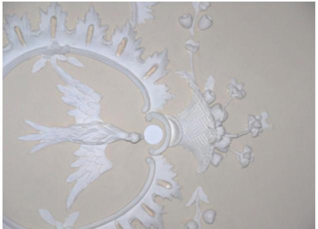
*Fig. 7 Circular concealed sprinkler head beside the bird's beak on a decorative plaster ceiling.*
