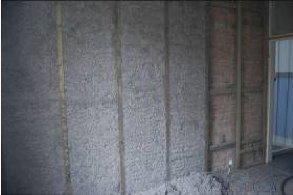
Fig. 5. Cellulose fibre trimmed finished flush prior to sheeting with plasterboard
