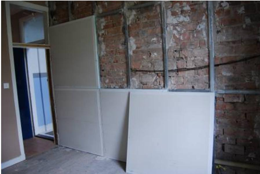
Fig. 7. Aerogel insulated board being applied to mass masonry on metal straps
