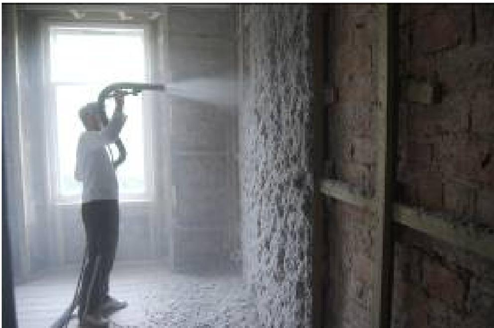
Fig. 4. Blown cellulose material sprayed damp directly onto masonry
