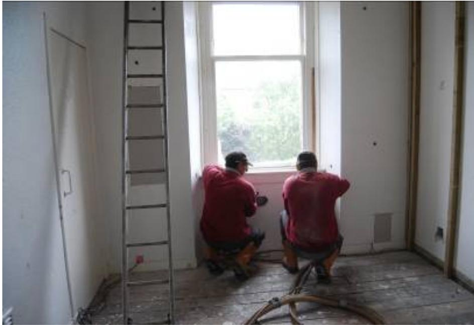
Fig. 3. Blowing bonded polystyrene bead behind existing wall lining
