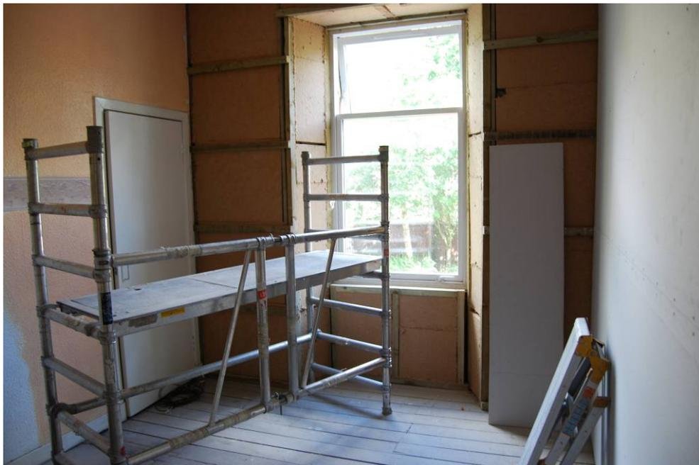
Fig. 6. Hemp board insulation applied between timber framing
