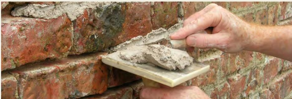
*Fig. 10: Joints should be well raked out and dampened before repointing work takes place.*
