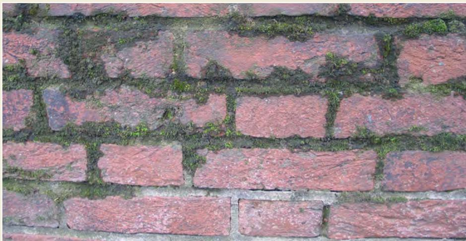
*Fig. 5: The presence of biological growth on brickwork is generally an indication of excess moisture from a building defect.*
