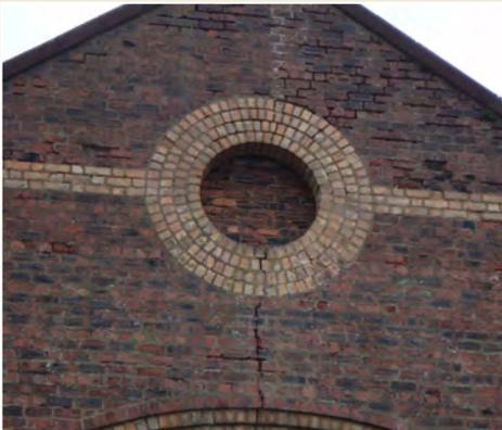
*Fig.4: Cracking is the most common sign of structural problems. A careful assessment of the cause and likelihood of further movement should be made in such circumstances.*
