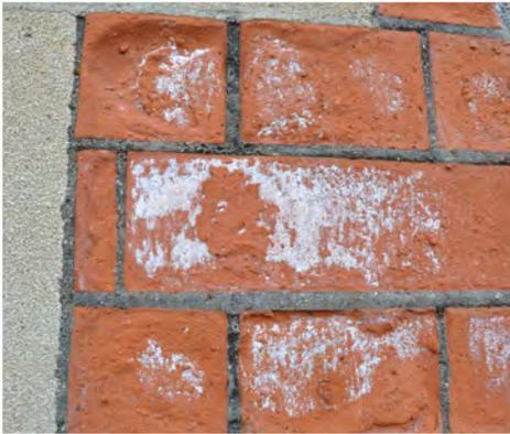
*Fig. 3: The presence of salts within brickwork is most commonly seen by a white residue on the surface of the brick.*
