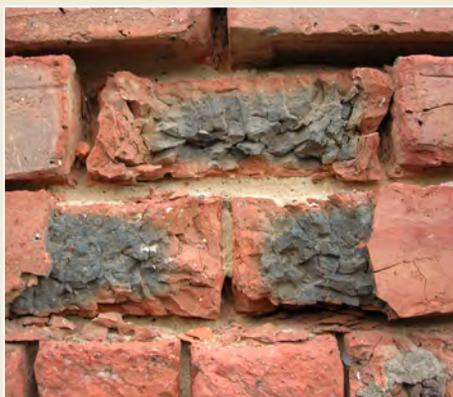
*Fig. 6: Where bricks have spalled, cutting out and replacing will often be the most appropriate repair technique.*
