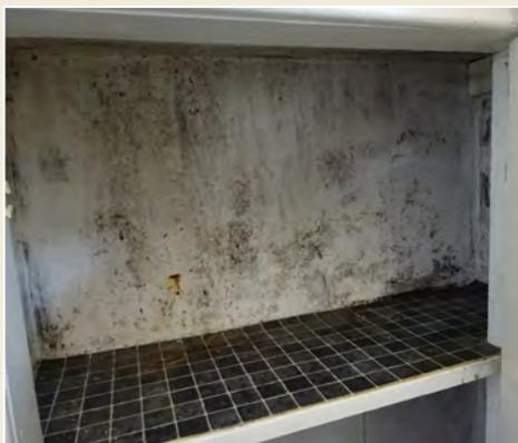
*Fig. 6 Mould growth in an unventilated press cupboard.*
