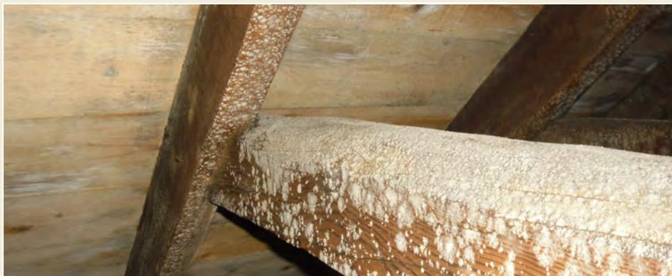
*Fig. 4 The positioning of mechanical extract ventilation is extremely important. Here moisture from a bathroom escaped into a roof space, causing a localised concentration of moisture, mould growth and timber decay.*
