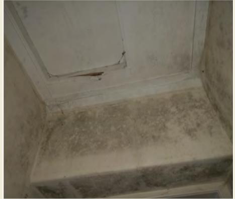
*Fig. 8 A cold spot has been created around this uninsulated loft access hatch, leading to mould growth.*
