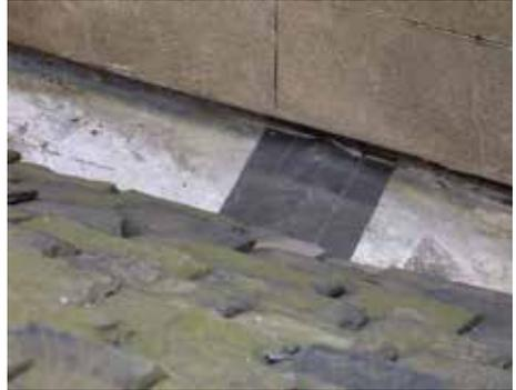
*Fig. 8 Temporary repairs such as this offer a measure of short term protection, but will not be as durable in the long term as those executed in lead.*
