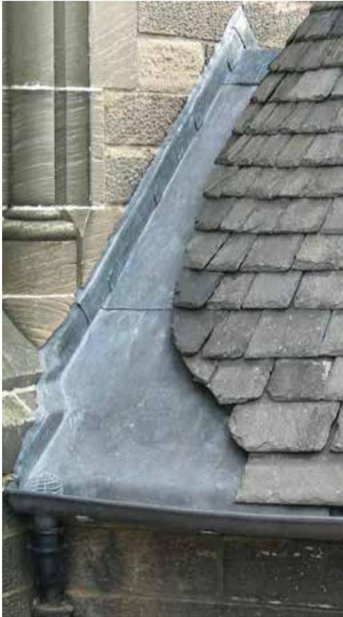
*Fig. 3* Lead is a durable material to use where a slate roof meets masonry such as at this skew cope.
