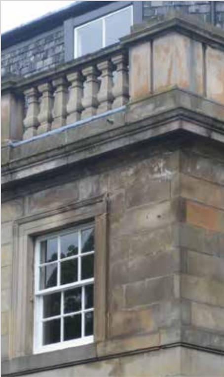
**Fig. 7** A blocked or leaking lead parapet gutter is causing saturation of the masonry below, seen here as the darker coloured stone and salt staining on the corner by the window.
