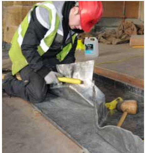
*Fig. 9 Fitting new lead sheet using traditional dressing techniques and tools.*
