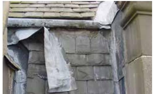
*Fig. 6 Wind uplift on exposed leadwork can result in the lead coming off.*
