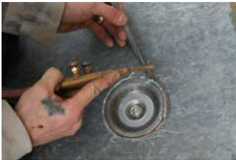
*Fig. 10 The use of additional fixings can be an effective deterrent against lead theft.*
