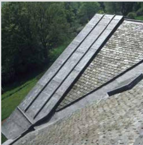
*Fig. 1 Lead is used extensively in this building as both a flat and pitched roof covering and to cover pediments and ridges.*
