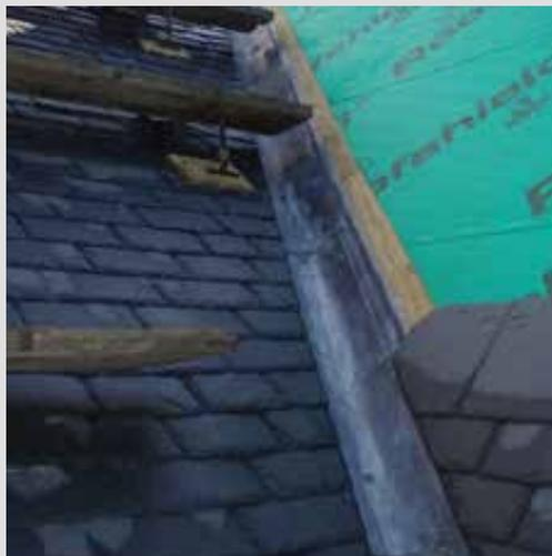
*Fig. 2 Lead is often used to protect areas of a roof where water is concentrated such as this valley gutter.*
