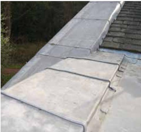
*Fig. 5 Milled lead sheet used to cover a flat roof.*
