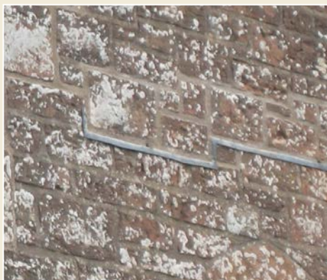
Fig. 7 Lead trays in the mortar to direct water away from the masonry.
