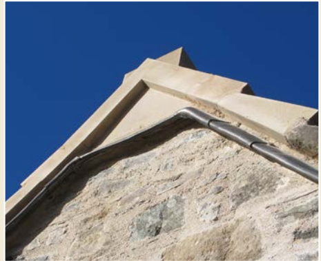
Fig. 11 Lead drip under a skew cope, angled to shed water (Photo credit: Jonathan Gotelee Architects).
