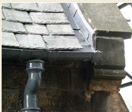
Fig. 14 A reworked skew junction with lead watergate.
