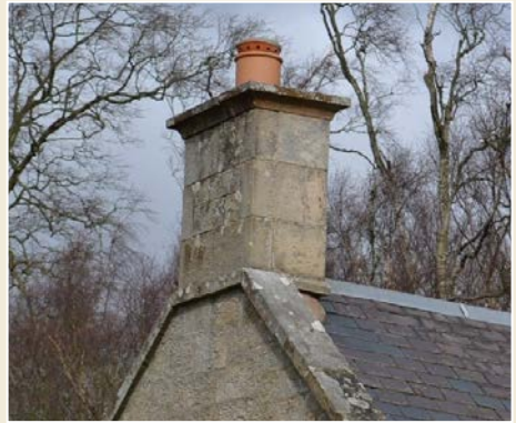
Fig. 10 Well detailed overhanging copes or 'tabling', and ceramic chimney cap.
