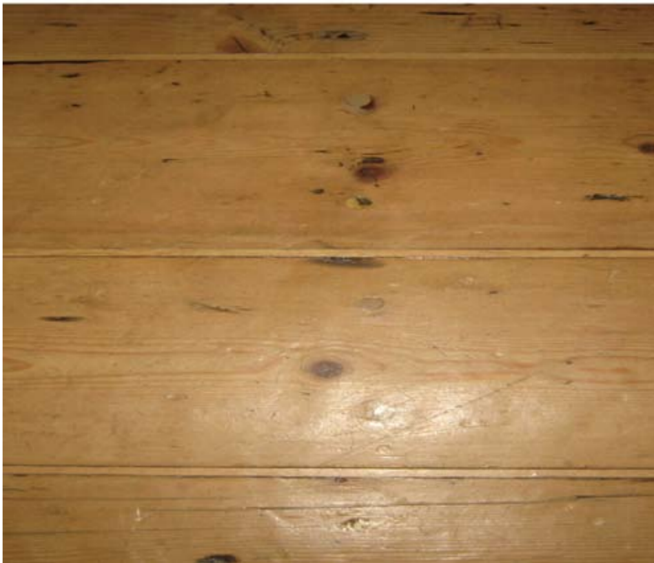
Softwood strips inserted where gaps are continuous
