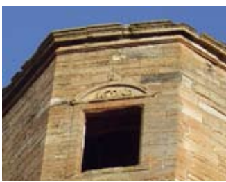
Date on north range
