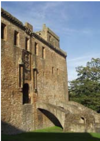
East range from the outside
