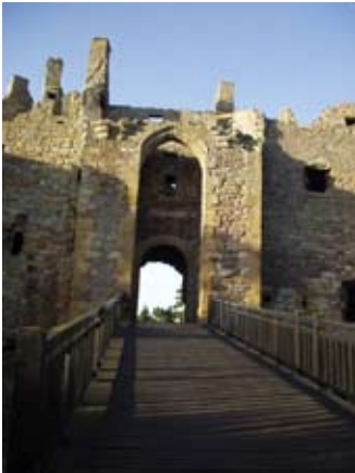
Bridge and Gatehouse
