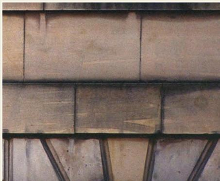
*Fig. 10: Stone indents painted in an attempt to blend in to the adjacent masonry.*
