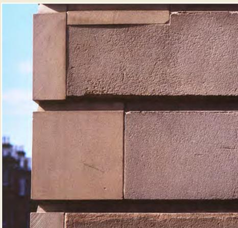
*Fig. 5: Ill-fitting replacement stones in the top corner. Circular saw marks can also be seen on the stone faces.*
