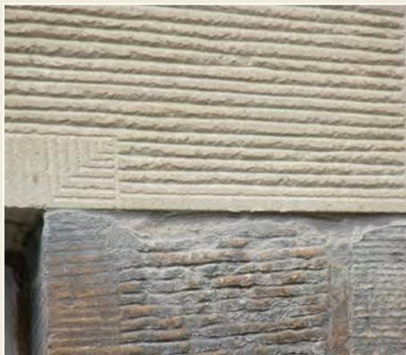
*Fig. 7: Damage to existing masonry caused during indenting.*
