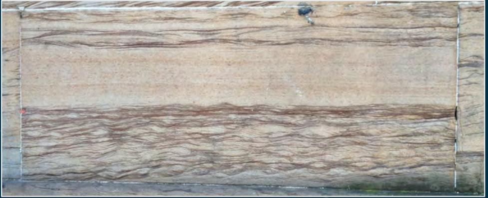
*Fig. 1: Visible bedding planes in this sandstone ashlar.*
