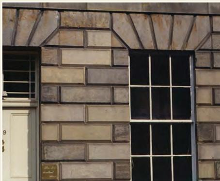
*Fig. 9: Successful ashlar indents that are 'weathering down' and blending in with the original masonry.*
