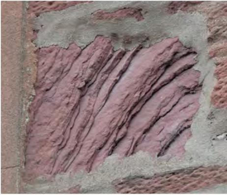
*Fig. 2: Face bedded sandstone, pointed with cement mortar, exhibiting delamination.*
