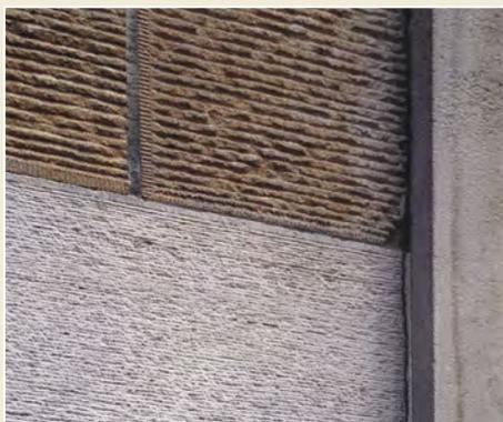
*Fig. 8: Variations in tooling due to differences in stone properties. It was not possible to tool the coarser grained replacement stone to the same fine detail as the original stone.*
