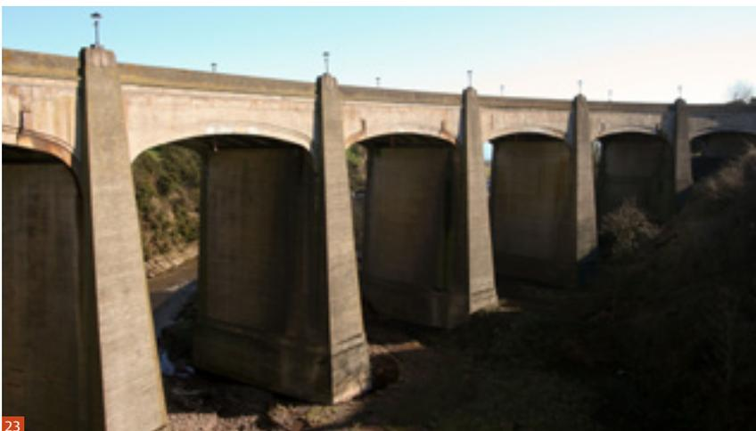
**Fig. 23** Reinforced concrete Bervie Jubilee Bridge, Aberdeenshire, built 1935. Impressed-current cathode protection system used to protect the bottom section of the main supporting beams.
