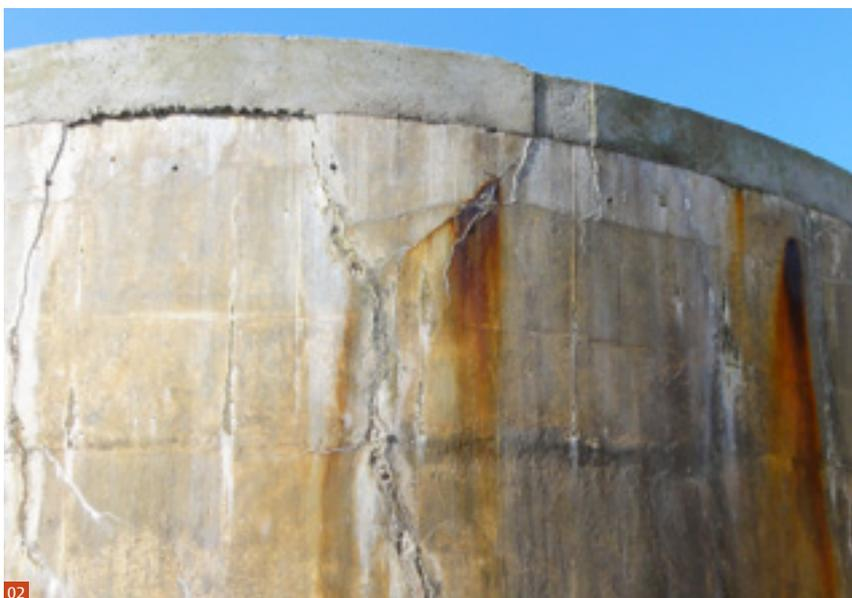
**Fig. 2** Rust stains on poorly repaired historic concrete. The stains in this case may be due to the presence of ferrous metal underneath the repair.
