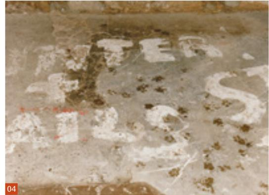
Fig. 3 The dark soiling is algal growth as a result of water run-off from a faulty sill and is unrelated to the shrinkage crack.
