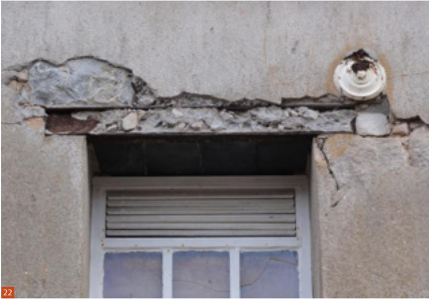
**Fig. 22** Disruption to concrete from corroding and delaminating wrought iron lintel (c. 1870s).
