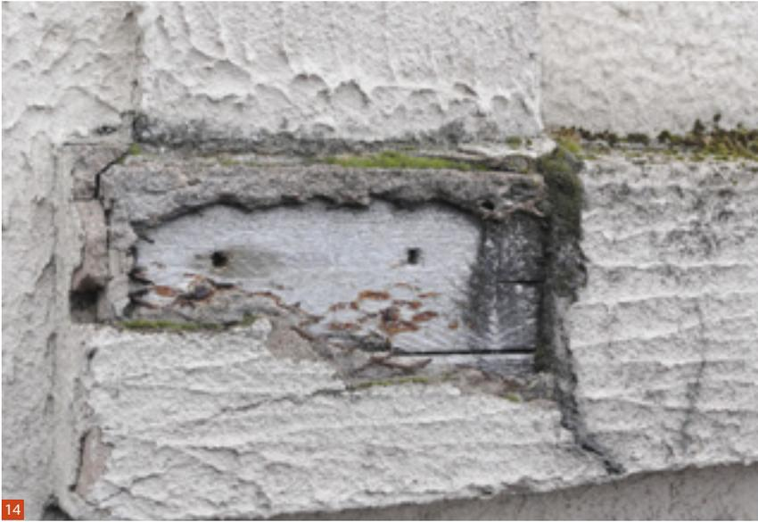
**Fig. 14** An extreme example of unsuitable repair to c. 1875 concrete. A softwood insert, covered with expanded metal lath and cement render, was used to replace deteriorating concrete.
