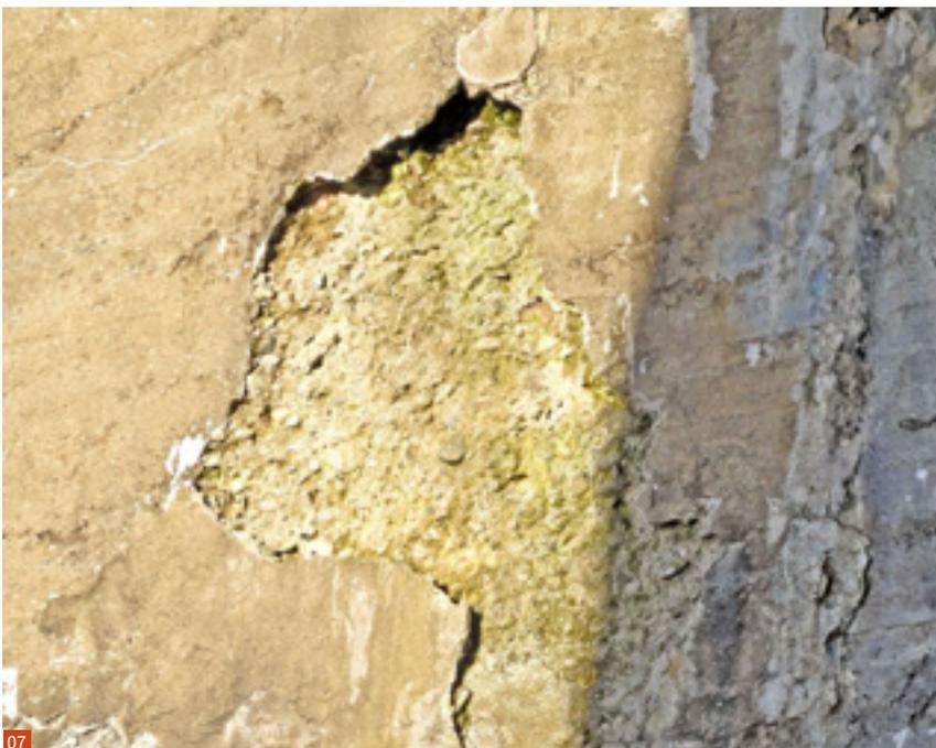
**Fig. 7** Concrete deterioration as a result of water penetration through shrinkage cracks with subsequent freeze-thaw cycles causing surface disruption. A patch repair would be suitable in this case.
