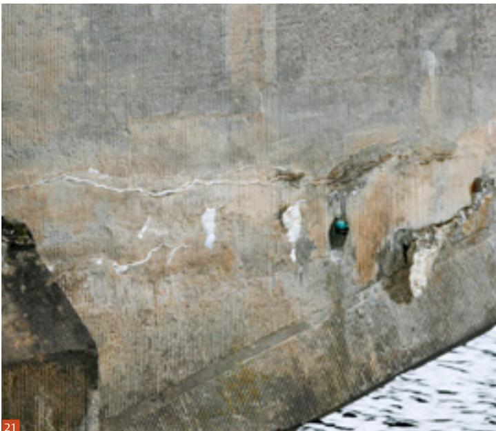
**Fig. 21** Chemical grouting of cracks in a reinforced concrete bridge. Note the indication that moisture is still present within the concrete.
