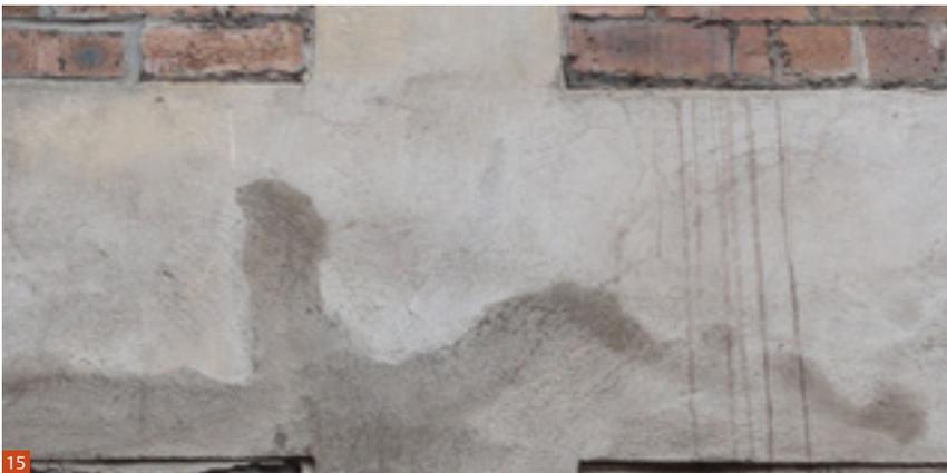
**Fig. 15** Surface repair to early 20th century reinforced concrete frame (Hennebique system).
