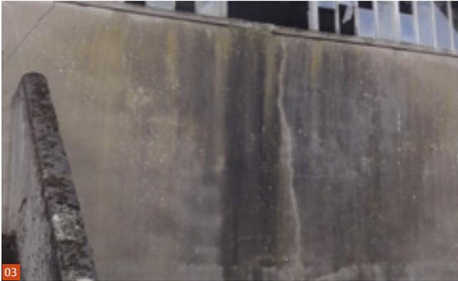
The algal growth shown in Fig. 3 is caused by water run-off due to a defective sill detail. There is no evidence of water damage or biological deterioration to the render, and it is not responsible for the shrinkage crack.
