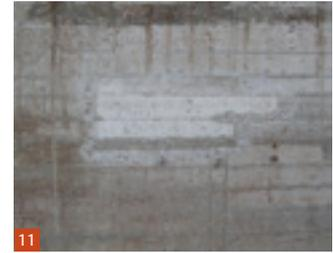
Fig. 11 Recent patch repair to historic mass concrete using formwork (shuttering) © Rowan Technologies Ltd.
