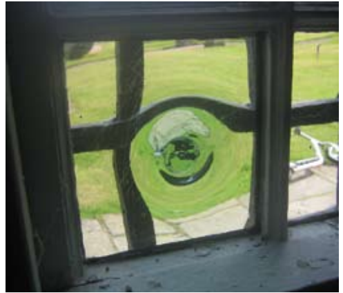
A "bull's eye" pane. This was the centre of the round table of crown glass and was the cheapest pane to be cut from the table. Image courtesy of R Curtis.
