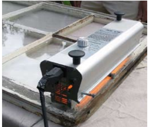
An infrared lamp in use
