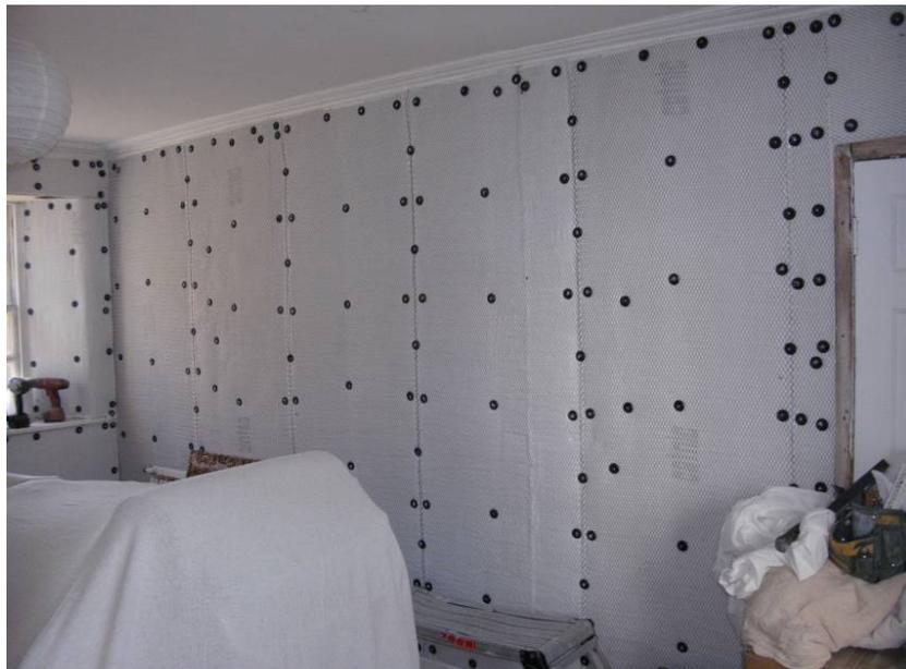
Fig. 2. Aerogel insulation applied as a blanket prior to application of a plaster finish
