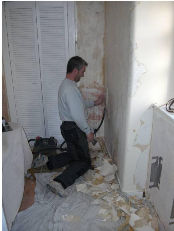
Fig. 3. Stripping of wallpaper and paint prior to application of calcium silicate board
