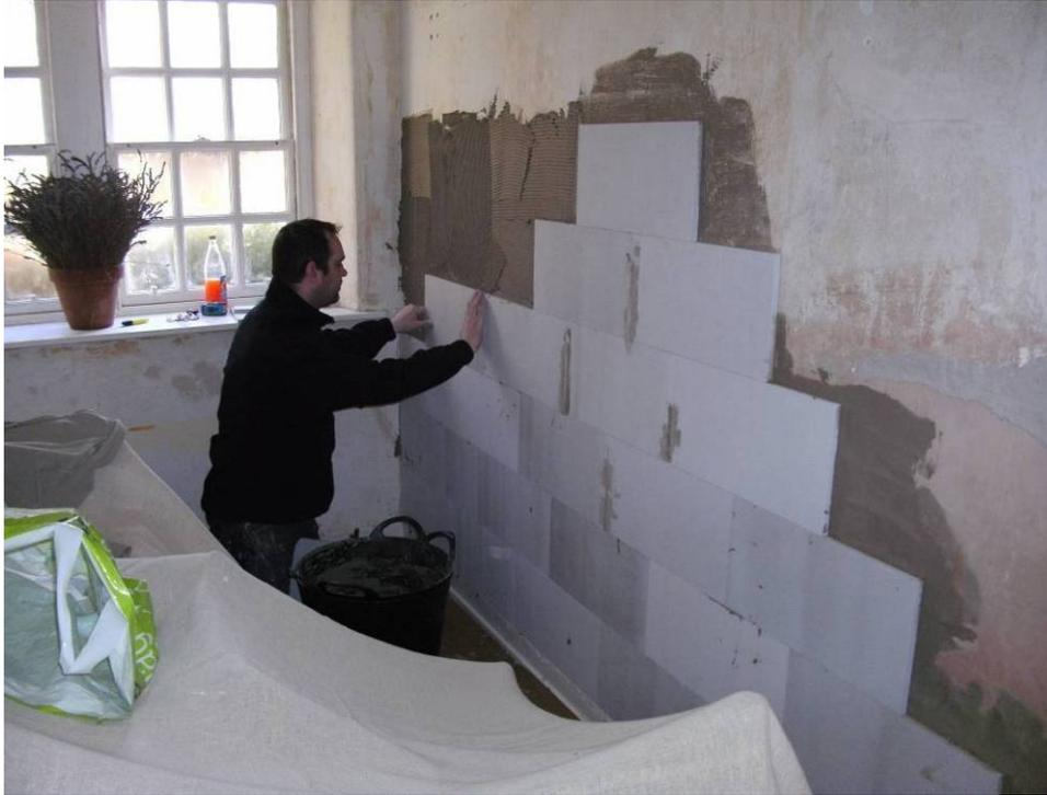
Fig. 4. Calcium silicate board being applied to a masonry wall at Wee Causeway
