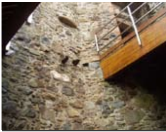
Roof beams in great hall
