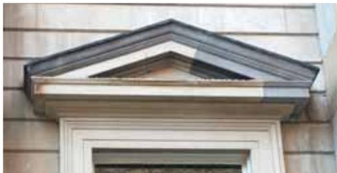
**Fig 16** This window pediment was repaired using a dark coloured sandstone to match the soiled building façade, prior to cleaning which has then lightened the adjacent masonry.
