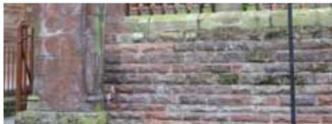
**Fig 9** Soiling from biological growth and salt accumulation due to water penetration.
