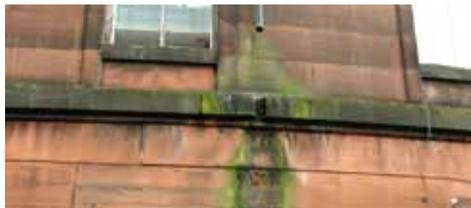
**Fig 7** Intense soiling and biological growth on masonry is typically directly associated with maintenance issues.
