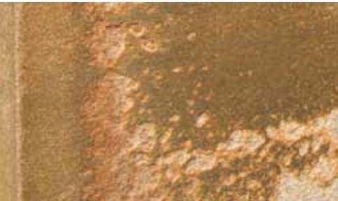
*Fig 4 Damage to a stable surface patina can expose weaker masonry underneath that is prone to decay.*
