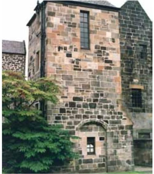
*Fig 5 An historic masonry building displaying variable soiling.*
