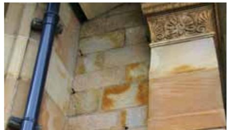
**Fig 12** Surface damage, bleaching and iron staining to stone masonry caused by inappropriate and aggressive stone cleaning.
