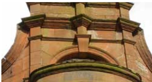
**Fig 20** Recently cleaned sandstone building showing relatively rapid recolonisation and biological soiling.
