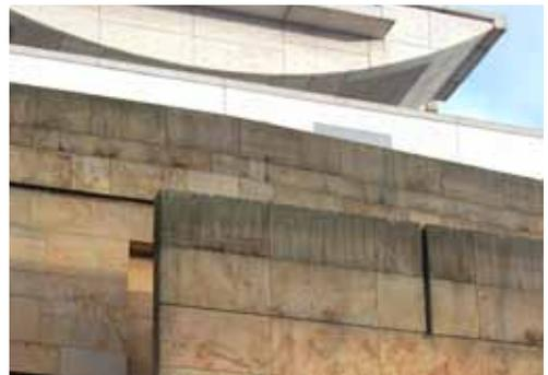
*Fig 3 New buildings will quickly exhibit soiling and a fresh appearance cannot be maintained forever.*
