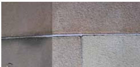
**Fig 18** Original soiled (left) and cleaned (right) sandstone masonry showing loss of the original smooth surface, resulting in a roughened texture which may be prone to resoiling and decay.
