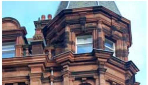
*Fig 6 Different surface finishes on stone masonry attract differing degrees of soiling which adds depth and richness to the building.*
