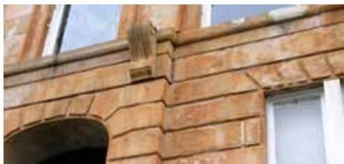
**Fig 17** Severely damaged stone façade following inappropriate cleaning, resulting in a loss of the external patination layer, discolouration from oxidation and increased deterioration.
