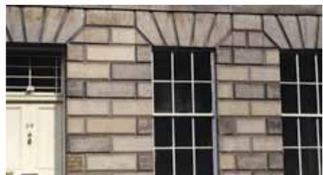
**Fig 14** Careful selection of replacement stone can ensure the new stone is visually in keeping with the original appearance of a façade.
