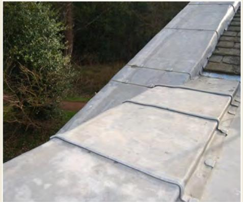
*Fig. 5: Milled lead sheet used to cover a flat roof.*
