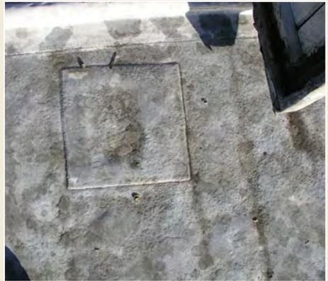
*Fig. 9: A patch repair with a piece of lead welded in place.*
