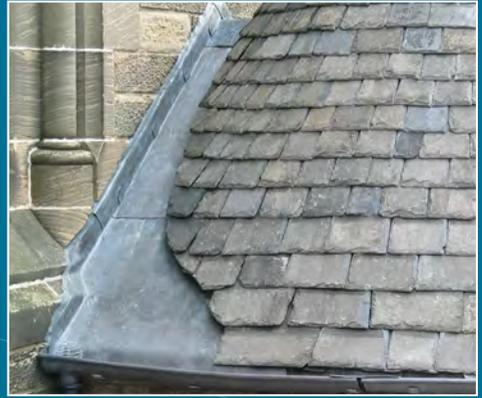
*Fig. 2: Lead is a durable material to use where a slate roof meets masonry, such as this abutment.*
