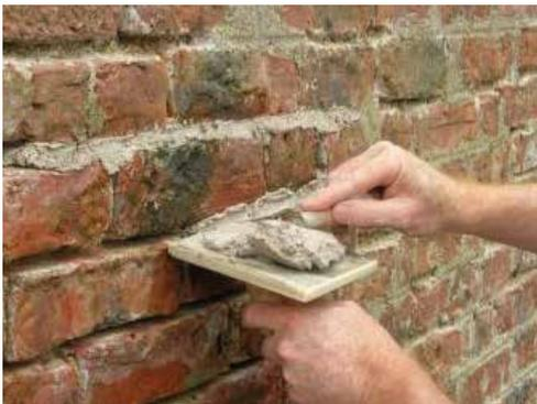
*Fig. 9 Joints should be well raked out and dampened before re-pointing work takes place.*
