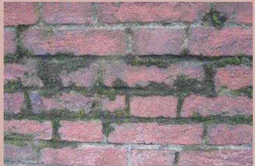
**Fig. 5** The presence of biological growth on brickwork is generally an indication of excess moisture from a building defect.
