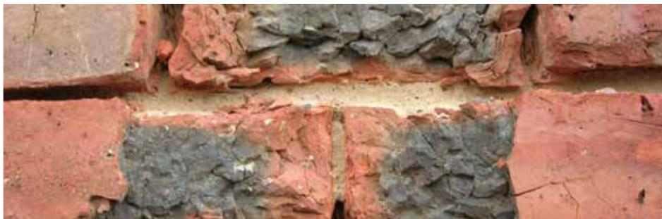
*Fig. 6 Where bricks have spalled, cutting out and replacement will often be the most appropriate repair technique.*
