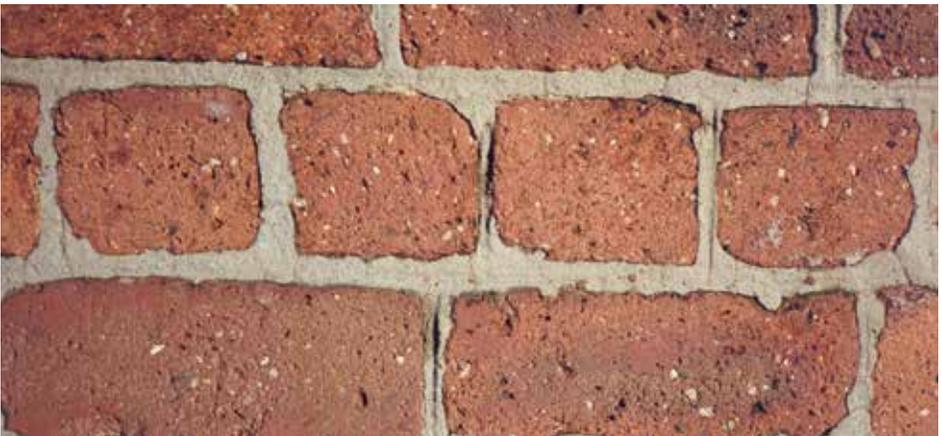
*Fig. 8B Brick after cleaning showing the potential damaging effects of abrasive cleaning methods. Note the loss of the protective external surface making the bricks more prone to decay.*
