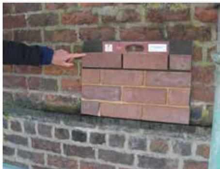
*Fig. 7 Replacement bricks should match those in situ as closely as possible, samples of bricks should be checked to gauge their suitability for a repair project.*
