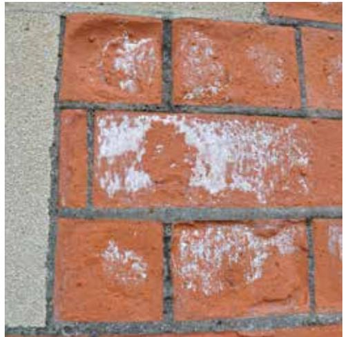
**Fig. 3** The presence of salts within brickwork is most commonly seen by a white residue on the surface of the brick.
