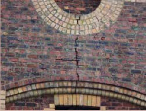
**Fig. 4** Cracking is the most common sign of structural problems. A careful assessment of the cause and likelihood of further movement should be made in such circumstances.
