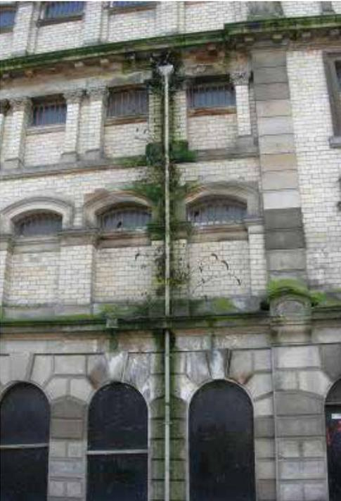
**Fig. 2** Water ingress from sources such as blocked gutters or downpipes is a major cause of deterioration of brickwork.
