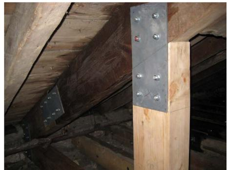
*Fig 8: Replacement of decayed timber*
