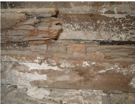
*Fig 7: Timber previously attacked by rot is particularly vulnerable to insect infestation*
