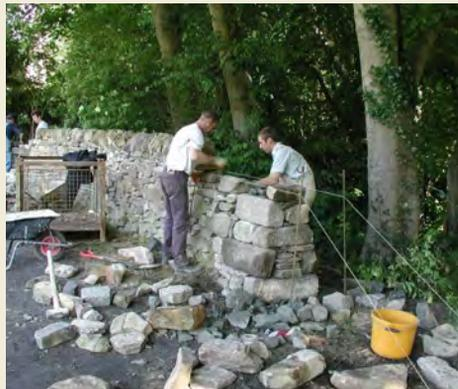
*Fig. 9: Rebuilding a section of a dry stone wall - note the construction of the wall-head.*
