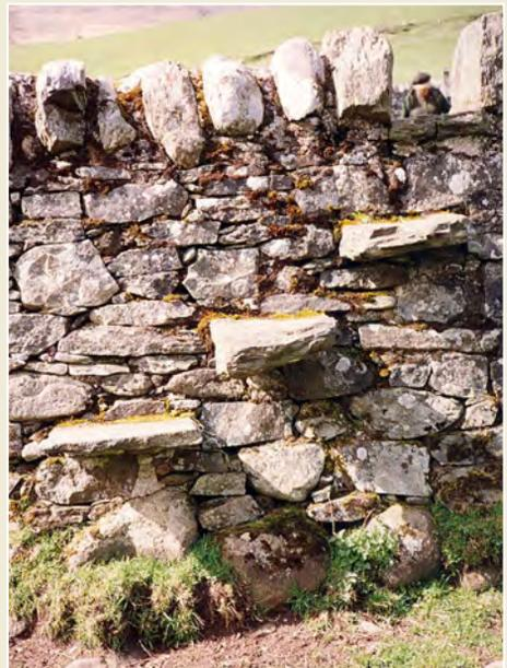
Fig. 7: Stiles built into dry stone wall.
