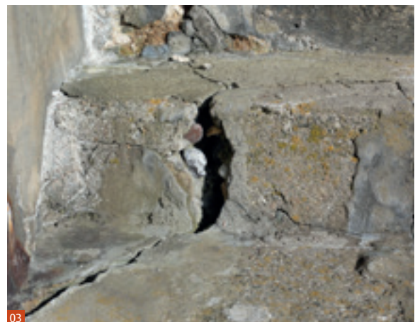
Fig. 3 The wall is poorly graded with large stones.
