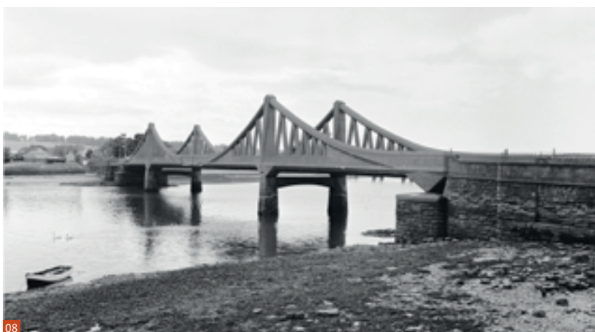
Fig. 8 Montrose Bridge, reinforced concrete cantilever construction. An unusual design for concrete construction (now demolished). SC 519533 © RCAHMS (Reproduced Courtesy of John R Hume). Licensor www.rcahms.gov.uk
