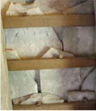
Roof tiles attached by pegs
