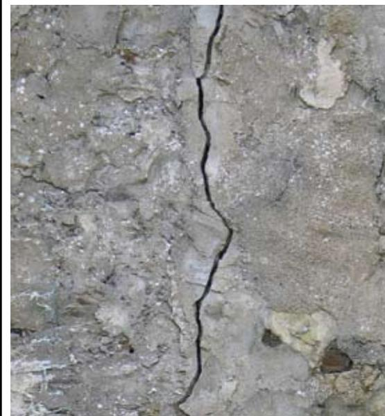
this width range, associated problems are also likely to emerge, perhaps requiring some localised replacement of fractured elements such as window sills, door lintels etc. Work may also be required to remedy any associated concerns regarding the weather-tightness of the building. This may have been compromised through disturbance to roof coverings or rainwater goods as a result of the movement.
