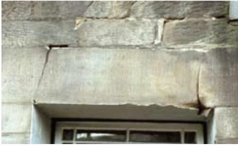
failure, particularly if the wall is also acting in a retaining capacity. Such crack patterns might also be found on parapet walls. These should be investigated at an early stage due to the added risk and safety problems that would be created if the parapet became loose and dislodged as a result of the structural failure, and the real risk that the crack could be allowing rainwater to enter the building interior.
