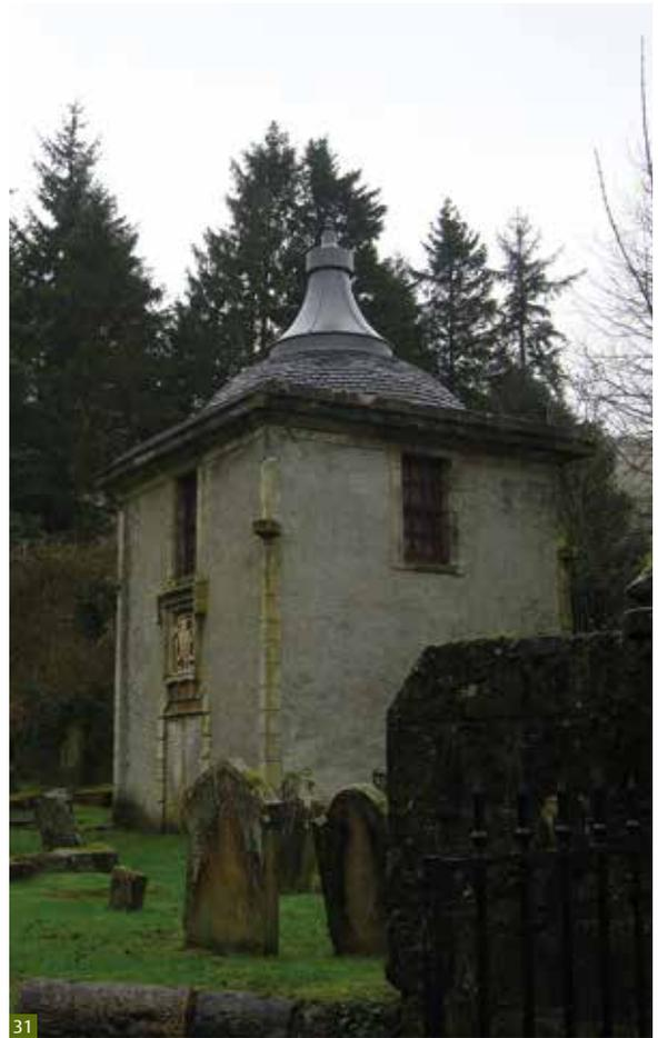
**Fig. 31** GRP cannot replicate the way lead looks, but may be an option for vulnerable and isolated structures.
