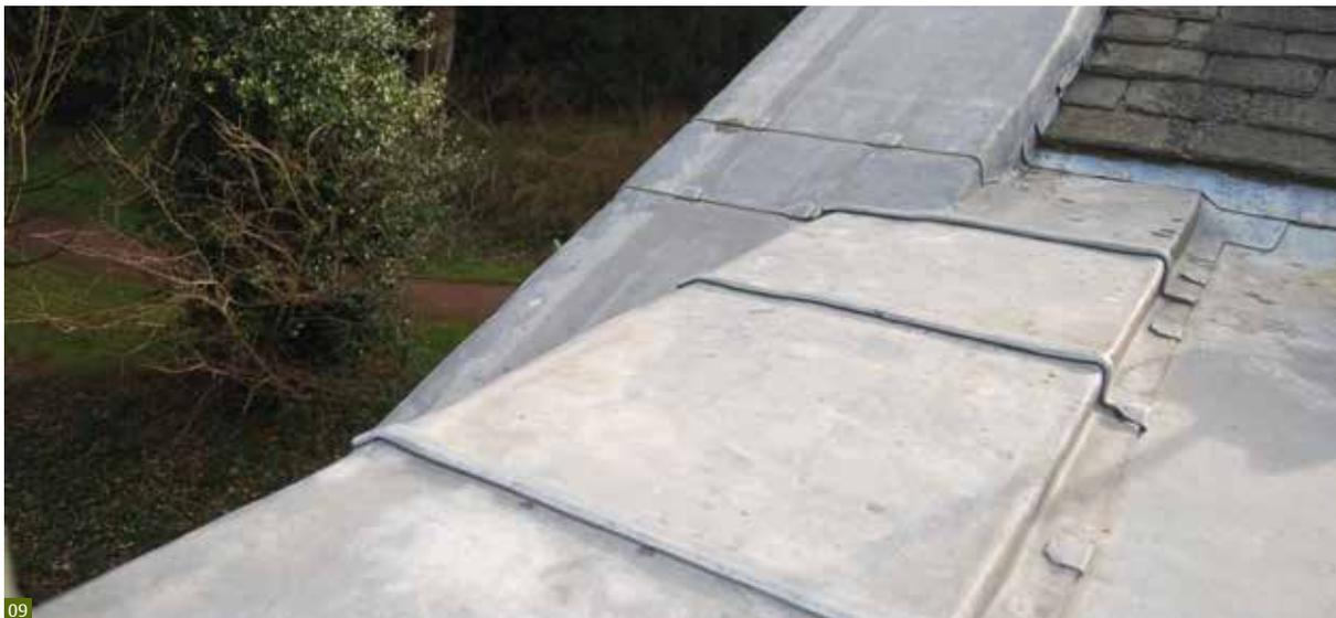
Fig. 9 Milled lead sheet.
