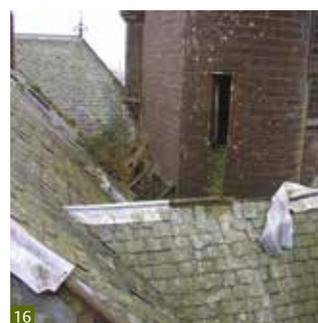
**Fig. 14** Damage to stonework and other building elements is a common complication where lead is stolen.
