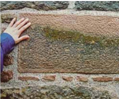
**Fig. 2** Inhibited biological growth due to alkaline conditions caused by new mortar.
