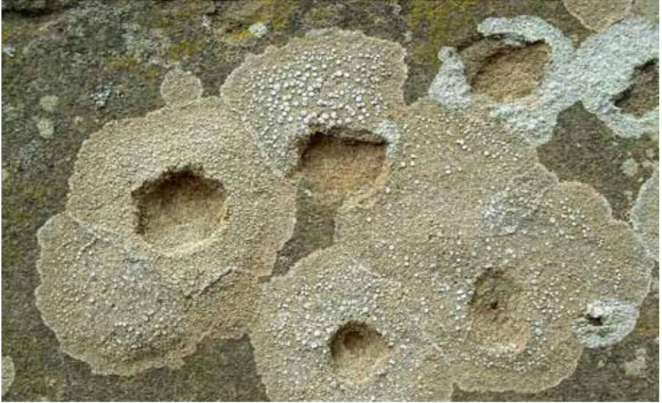
*Fig. 4 Rare example of damage to sandstone masonry caused by lichen growth.*
