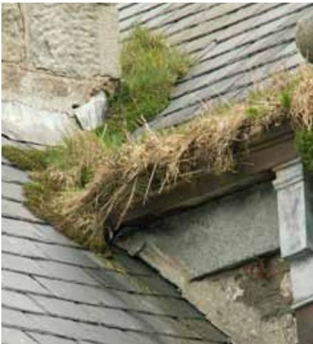
*Fig. 5 Guttering clogged by plant growth.*
