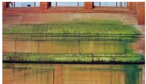
*Fig. 6 Rapid re-colonisation by algae of a recently cleaned sandstone building.*
