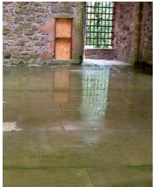
**Fig. 3** Slime producing algae may result in slippery surfaces.
