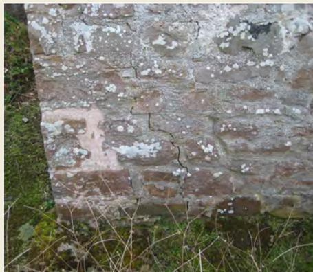
*Fig. 11: Cracks due to softer ground on a damp corner.*
