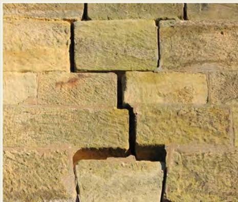
*Fig. 6: Very severe structural movement, requiring temporary support work.*
