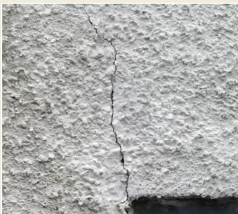
*Fig. 7: A fine hairline crack on a rendered façade, possibly caused by normal seasonal expansion and compression of the building materials*
