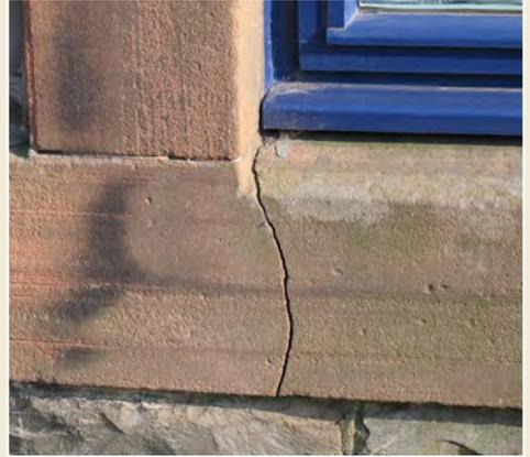
*Fig. 3: A thin crack on a window cill.*
