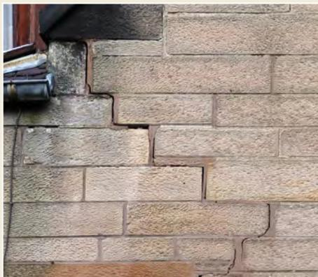
*Fig. 8: A stepped crack running diagonally.*
