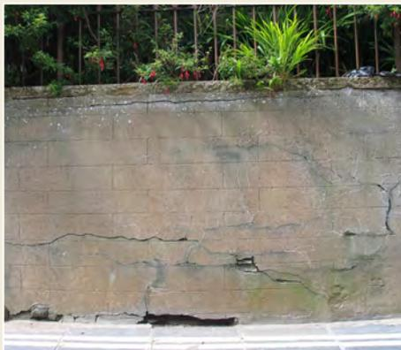
*Fig. 10: Cracks indicating outward pressure at the foot of the retaining wall, probably due to moisture retention behind the cement render.*
