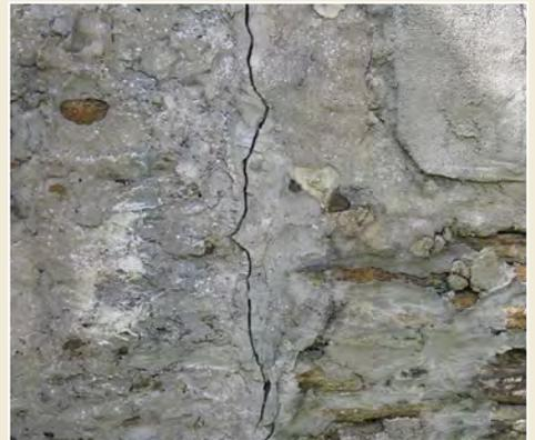
*Fig 4: A medium sized crack on a stone wall. This will need remedial work.*
