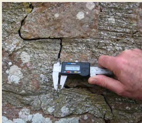
*Fig. 13: Using a micrometer to monitor a crack.*
