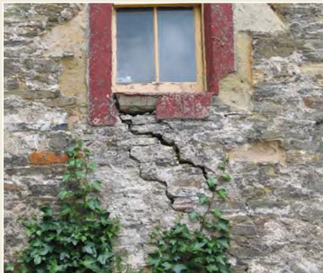
*Fig. 5: A severe crack, requiring professional advice and stabilisation.*
