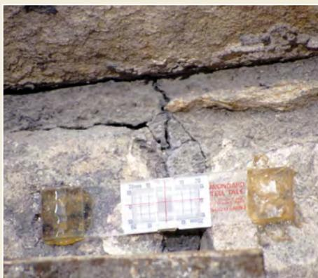
*Fig. 12: A tell-tale installed over a crack.*
