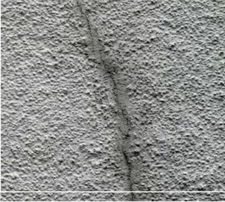
*Fig. 2: A hairline crack on a rendered wall.*
