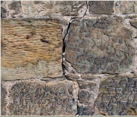
*Fig. 1: A typical crack in a traditional stone wall.*
