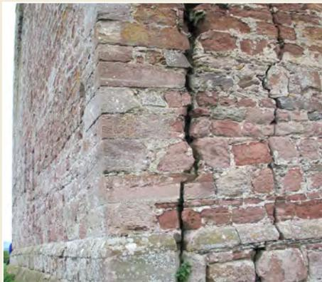
*Fig. 9: A vertical crack running through both, mortar joints and stones.*
