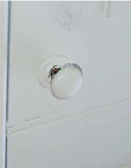
*Fig. 10* Painted timber shutter knob fitted to shutter's outer leaf.
