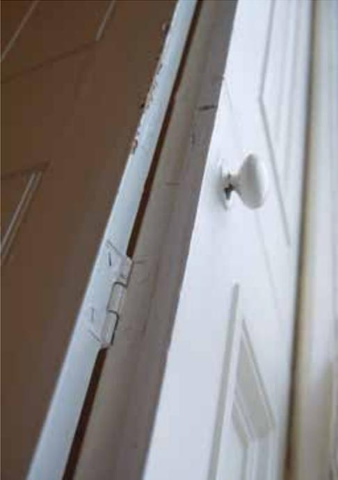
*Fig. 3* Shutter half open showing the outer panelled leaf and the middle leaf, with rebated joints to reduce light penetration when closed.
