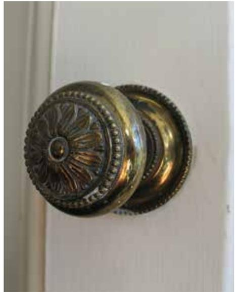
*Fig. 11* Brass shutter knob fitted to shutter's outer leaf.
