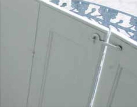
**Fig. 8** Small latch used to hold shutters in the closed position at the stiles.
