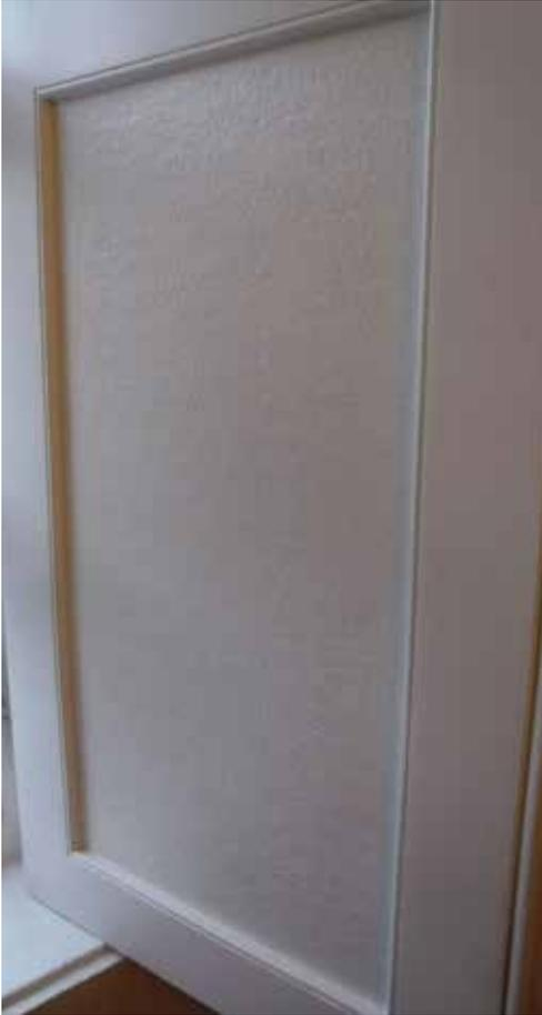
*Fig. 12 Newly instated insulated timber shutters.*
