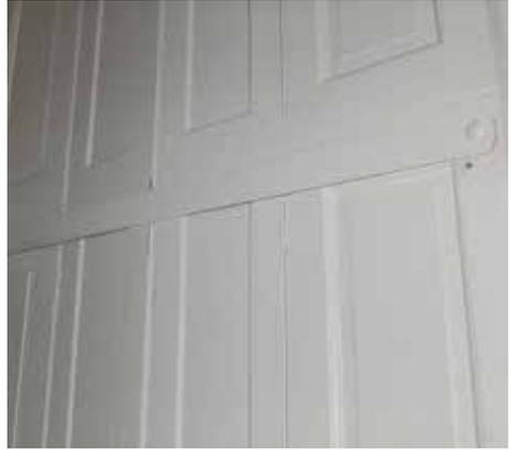
**Fig. 7** Iron stay bar in position, spanning the width of the window opening.
