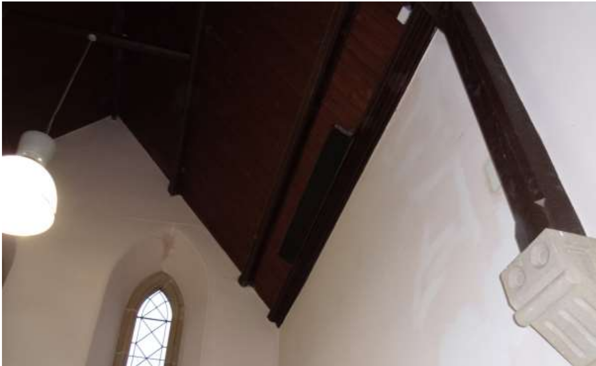
Fig. 4: The radiant panels visible middle right, just above wallhead level
